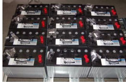
Deep cycle lead-acid batteries have proven to be one of the best (and most affordable) battery types for alternative energy system battery banks for these reasons:
